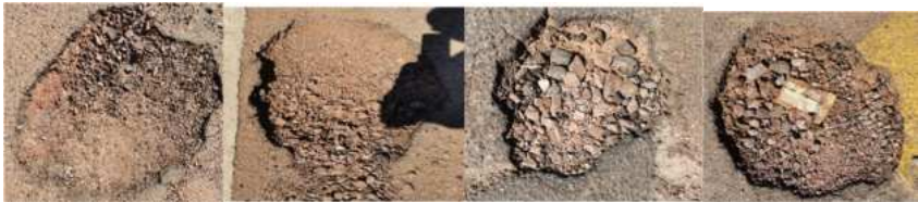
Potholes around the circle Krige/Brandwag there are about 50 potholes
